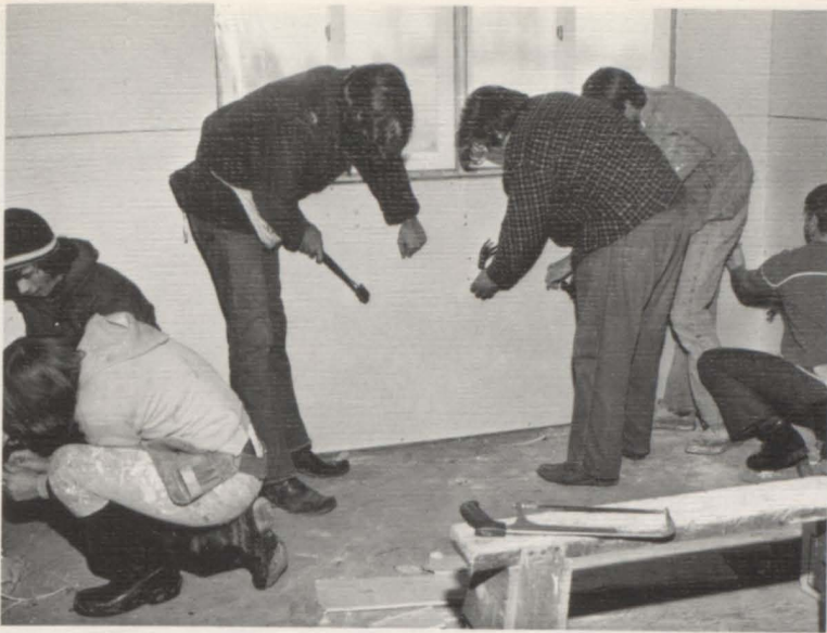
House being built by Building Trades class
